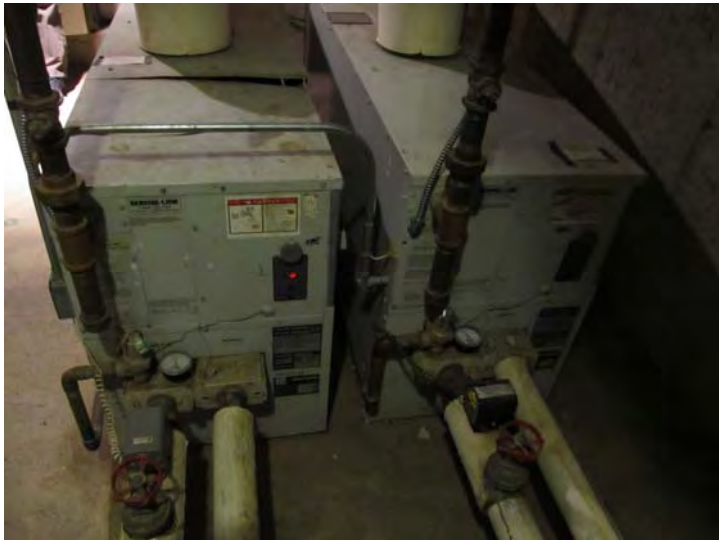
Lochinvar gas-fired boilers serving Units 1-19 are at or near end of expected useful service life
