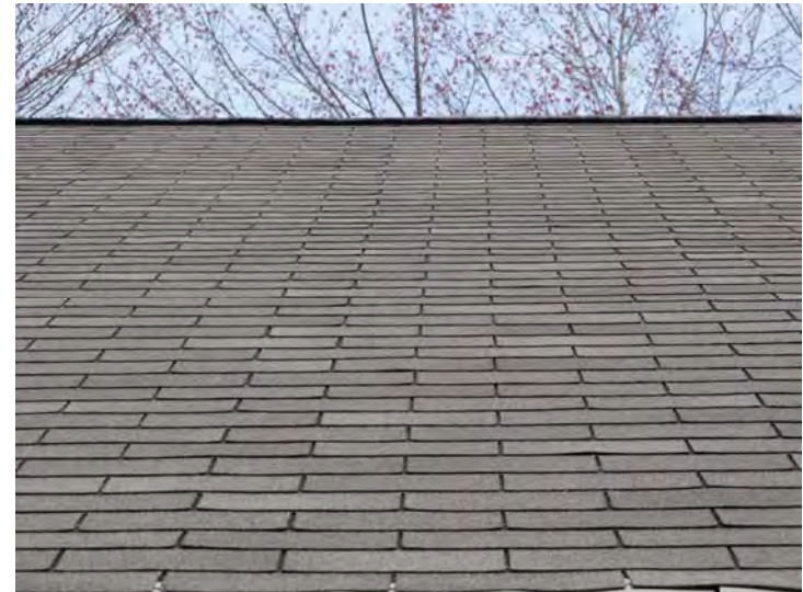
Both buildings have pitched roofs with newer three-tab shingle coverings – No problems noted
