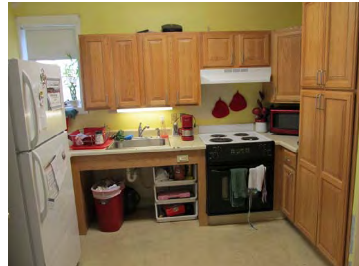
Typical handicap accessible unit kitchen – Note cabinetry design does not incorporate a thirty-inch wide work surface with knee clearance space
