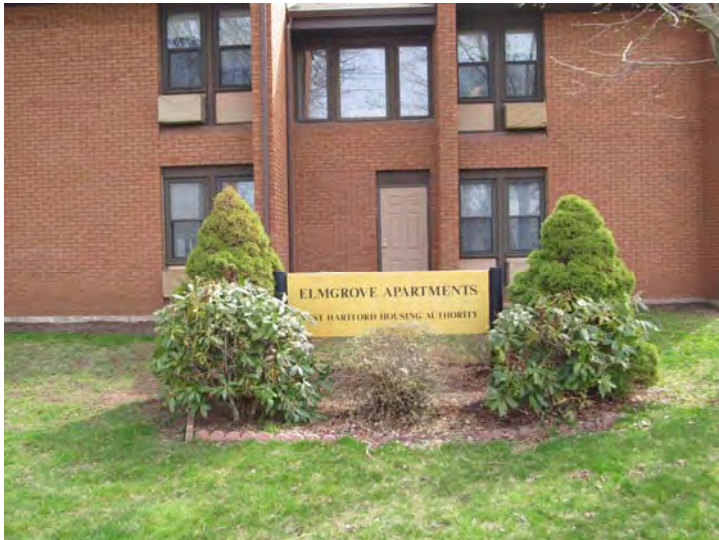
Unit windows were replaced in recent years – Common area (stairwell above door in center) windows are original to the development
