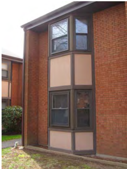
Brick veneer and wood siding/trim materials are all in generally good condition at the present time
