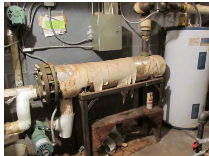
Original shell and tube and heat exchanger for domestic hot water production at Units 20-40
