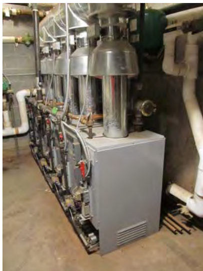
Newer Hydrotherm modular boiler plant for heat and domestic hot water generation at Units 20-40
