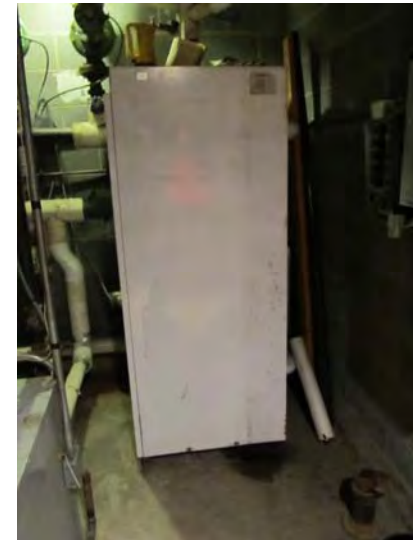
Triangle-Tube Phase III indirect-fired domestic hot water storage tank for Units 1-19
